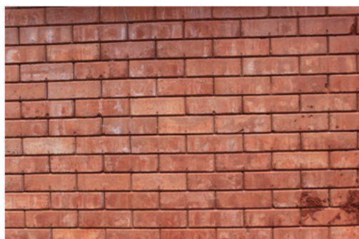
Figure 6. Masonry wall using compressed stabilized earth blocks
