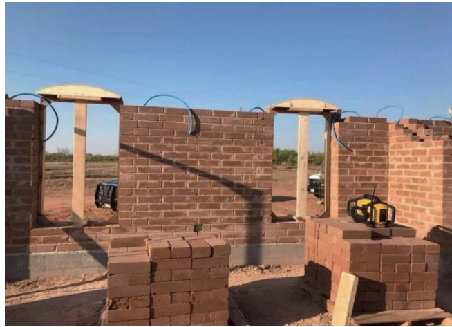
Figure 7. Construction of masonry wall using compressed stabilized earth blocks
